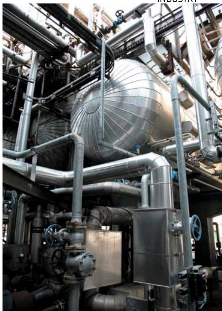
A REACTOR WITH DEDICATED EQUIPMENT, HORIZONTALLY POSITIONED. THIS TYPE OF INSTALLATION IS USED TO PERFORM CHEMICAL REACTIONS.
