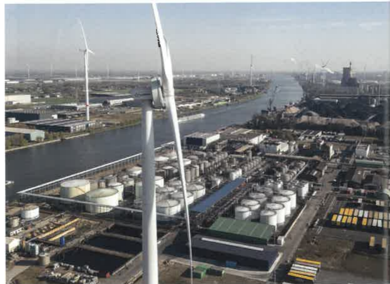
An on-site wind turbine and a partnership with the nearby Bio Energy Base biomass plant provide Gadot Belgium with renewable energy, already resulting in a 55% reduction in CO 2 emissions on the way to 100% renewable energy.
